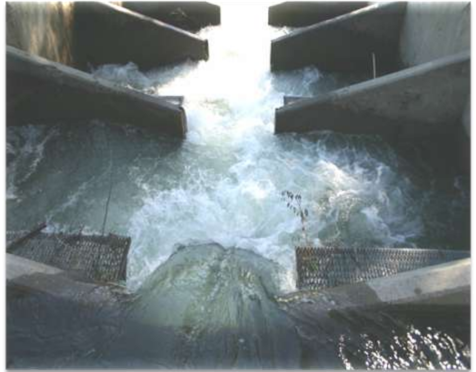
A typical fishway with steps
